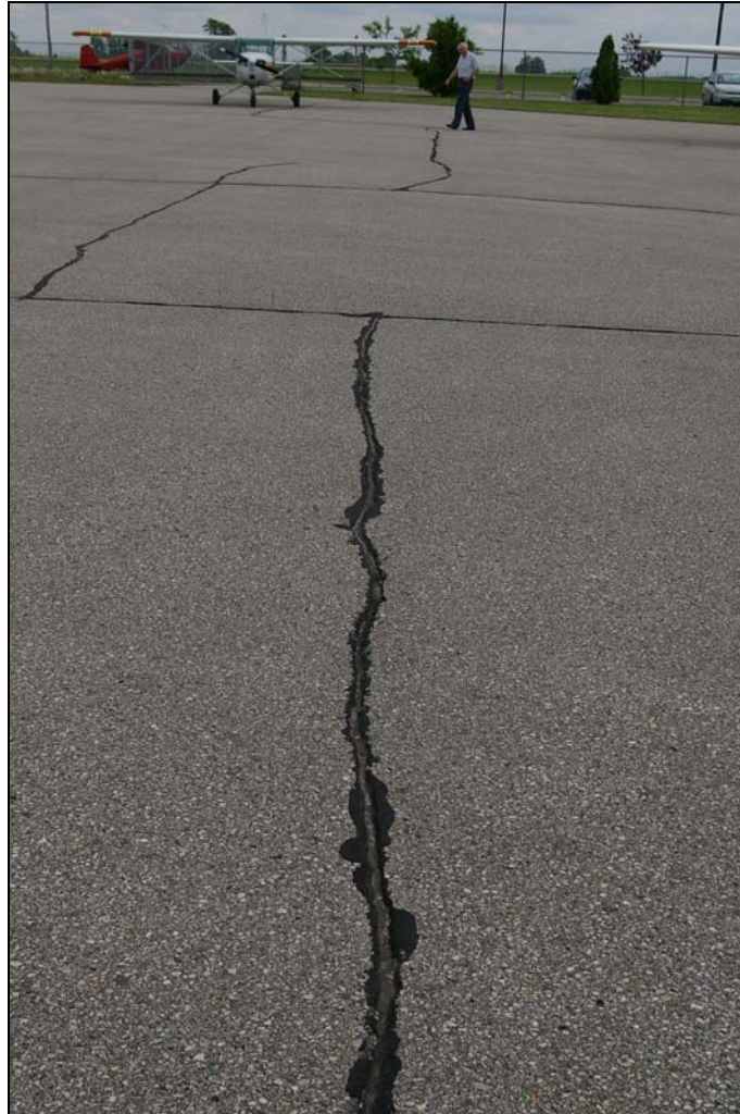
Photo 7: Typical condition of main Apron.
