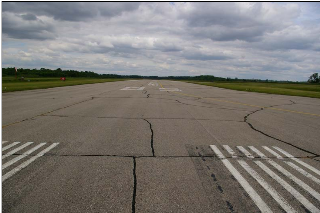
Photo 2: Typical condition of reconstructed portion of Runway 05-23 (1988 construction).
