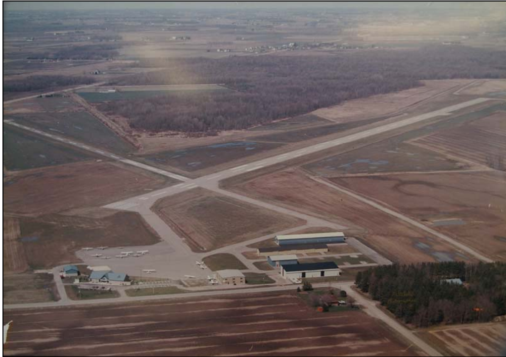
Photo 1: Overview of Airport
