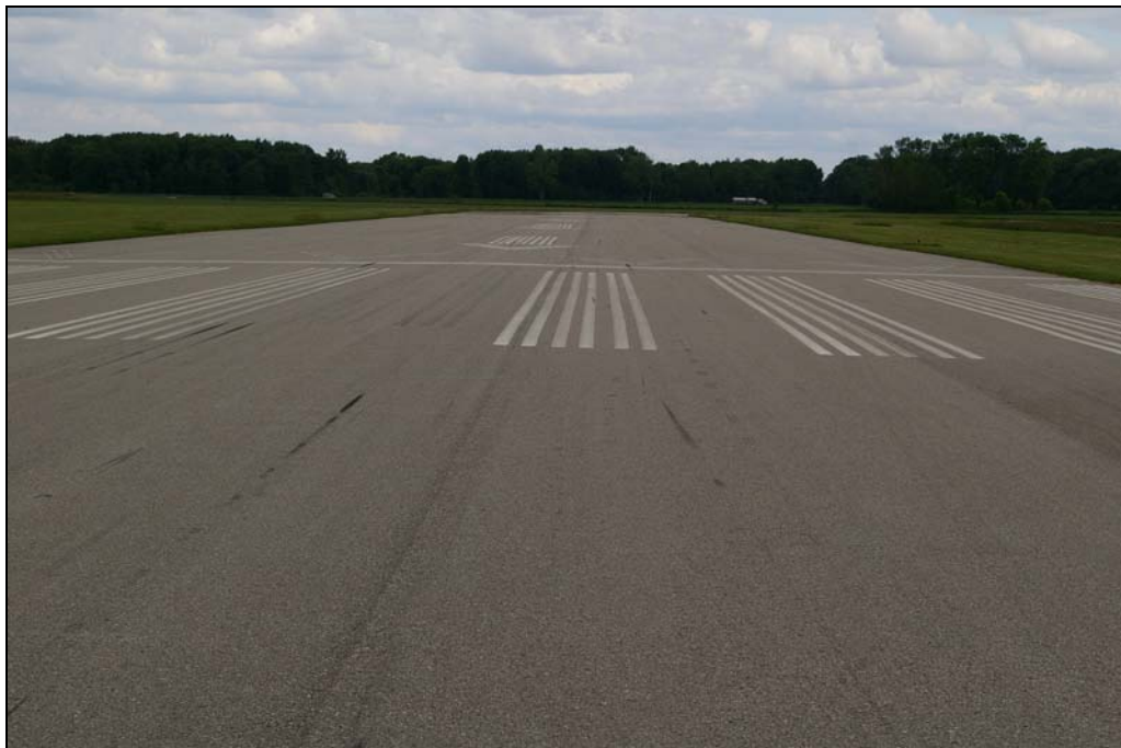
Photo 9: Typical condition of extension of Runway 05-23 (1993 construction).
