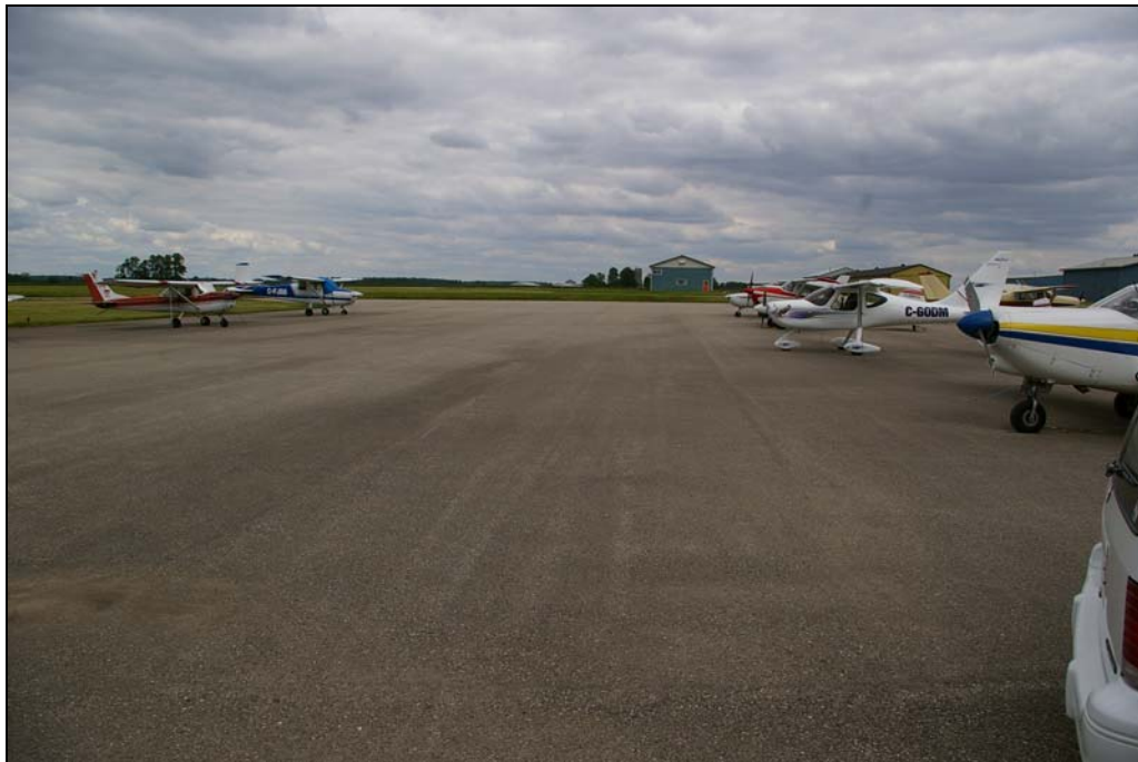
Photo 13: Typical condition of Apron Extension.
