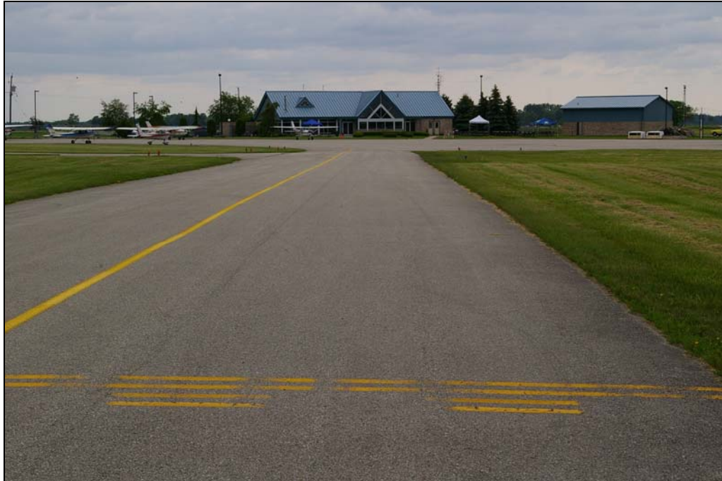
Photo 12: Typical condition of Taxiway B (E-W Portion).
