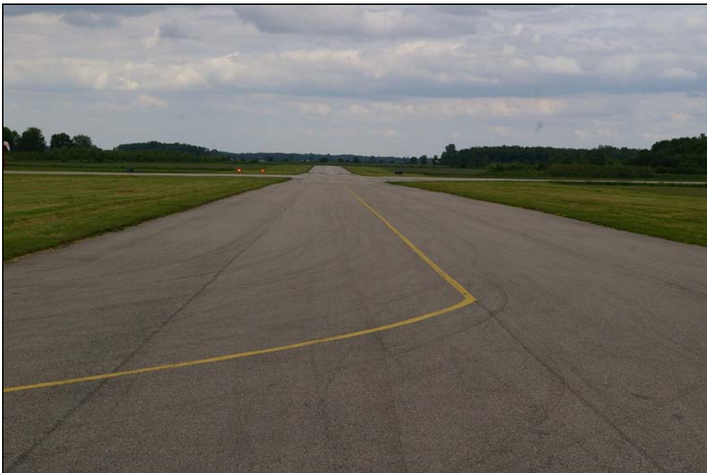
Photo 11: Typical condition of Taxiway B (abandoned Runway 17-35).
