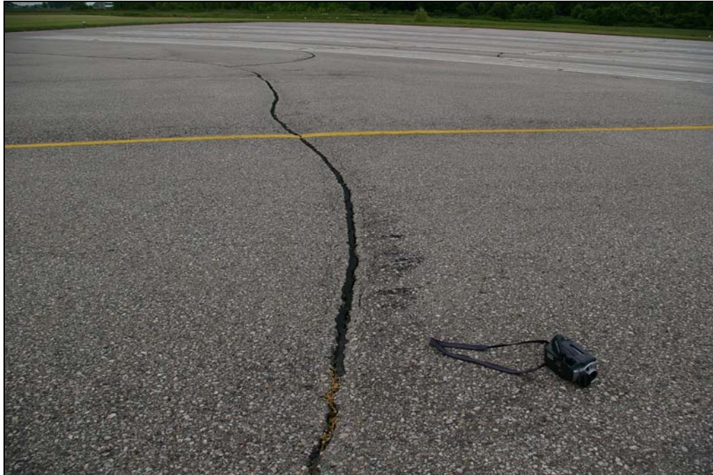
Photo 8: Typical condition of Taxiway A.
