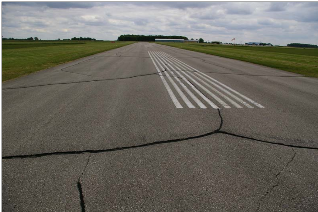
Photo 6: Typical condition of Runway 17-35 in the vicinity of intersection with Runway 05-23 (1988 construction).
